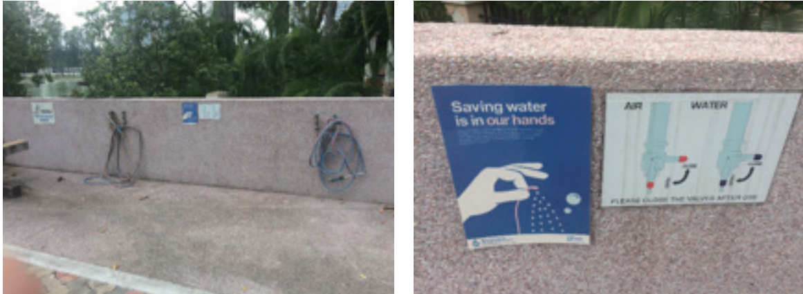
Figure 19 boat washing station - using water and air together to reduce water consumption
