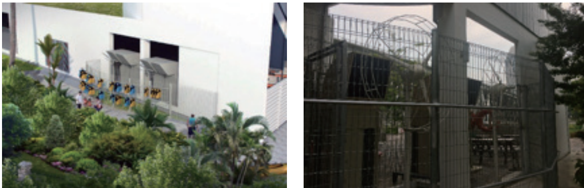
Figure 20 Compressor - Using wind from compressor to dry life jackets
